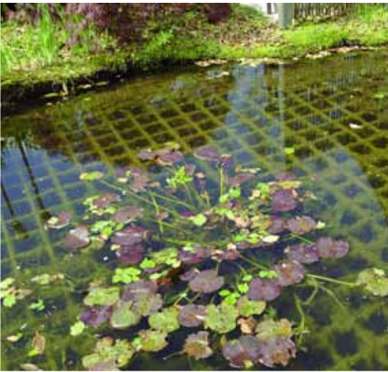
Et armeringsnet i vandet giver sikring.
